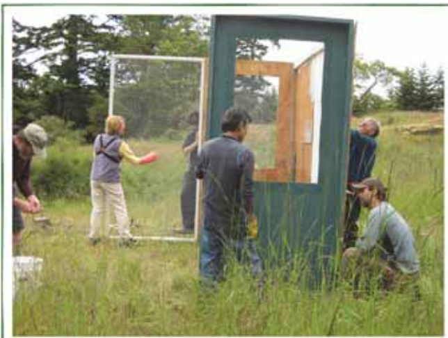
Constructing aviary © Gary Slater
